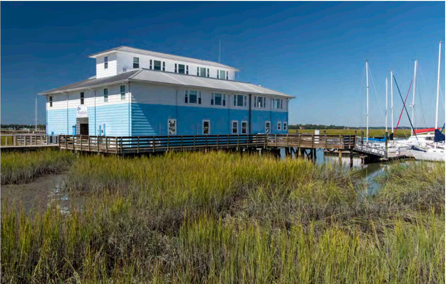
Photo source: Design Workshop
