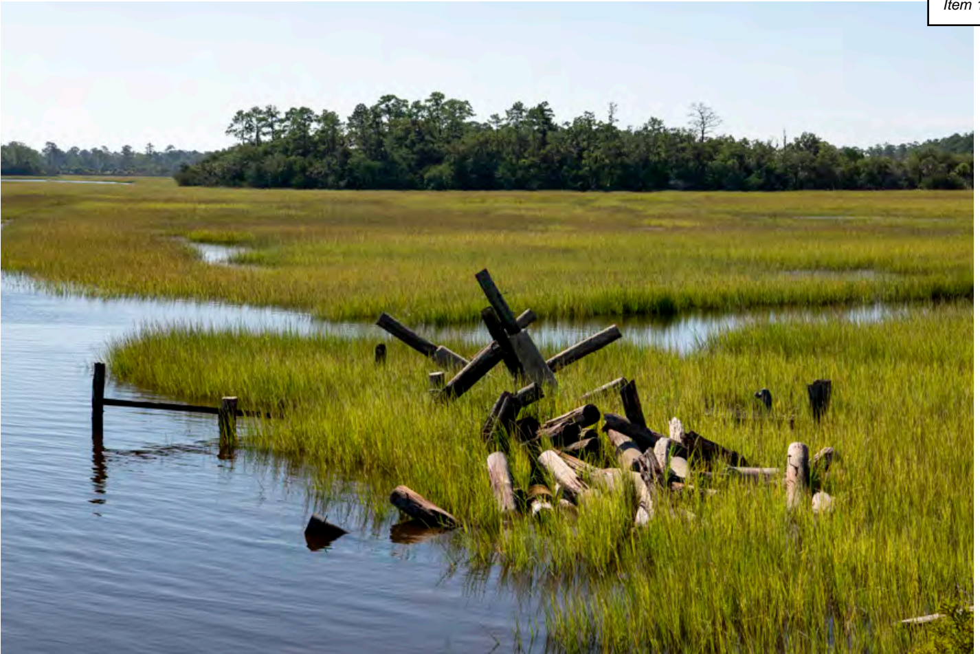
Photo source: Design Workshop
