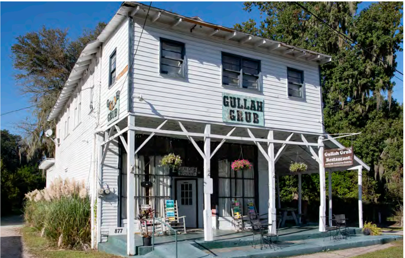
Photo source: Design Workshop
