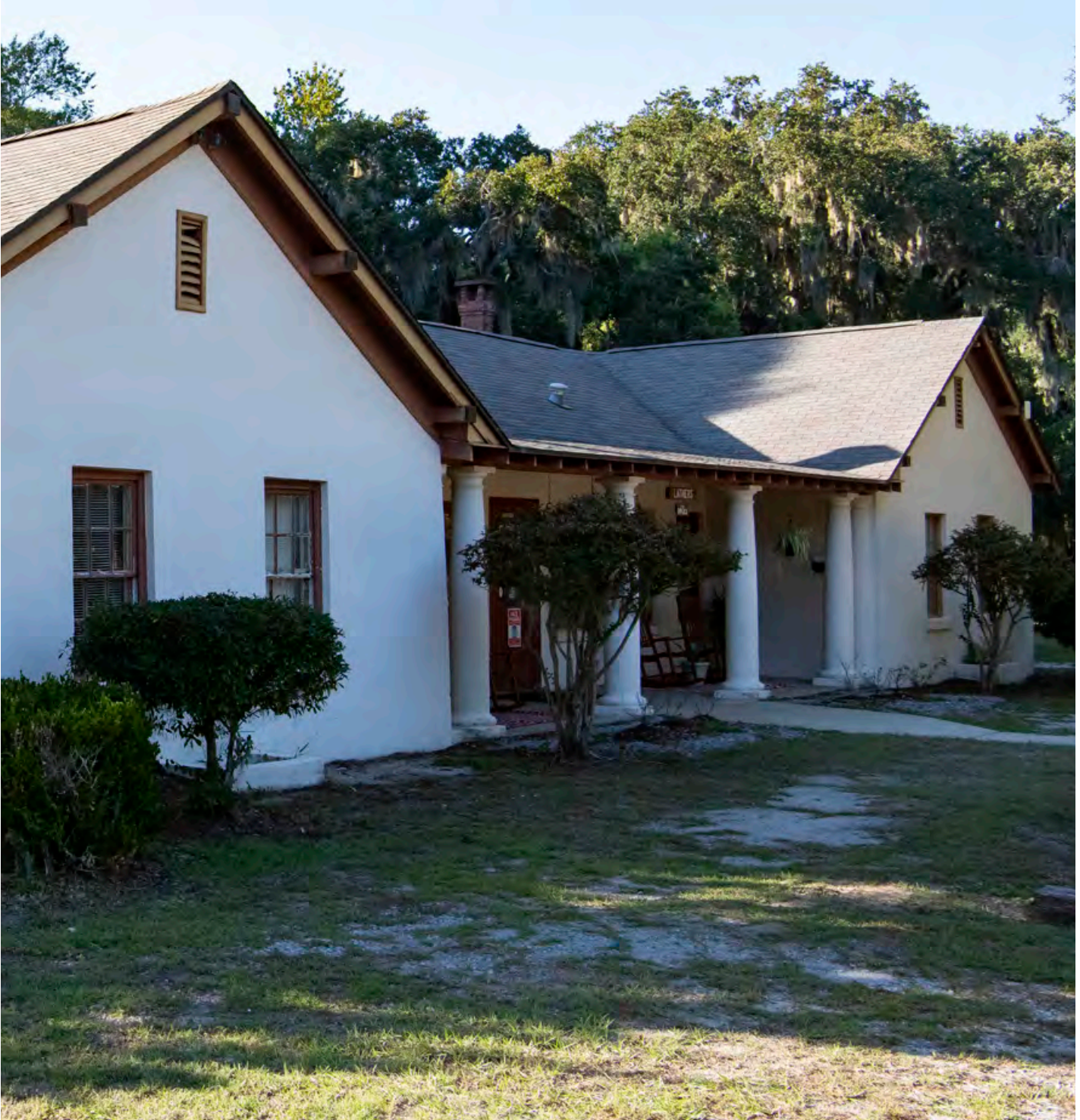
Photo source: Design Workshop
