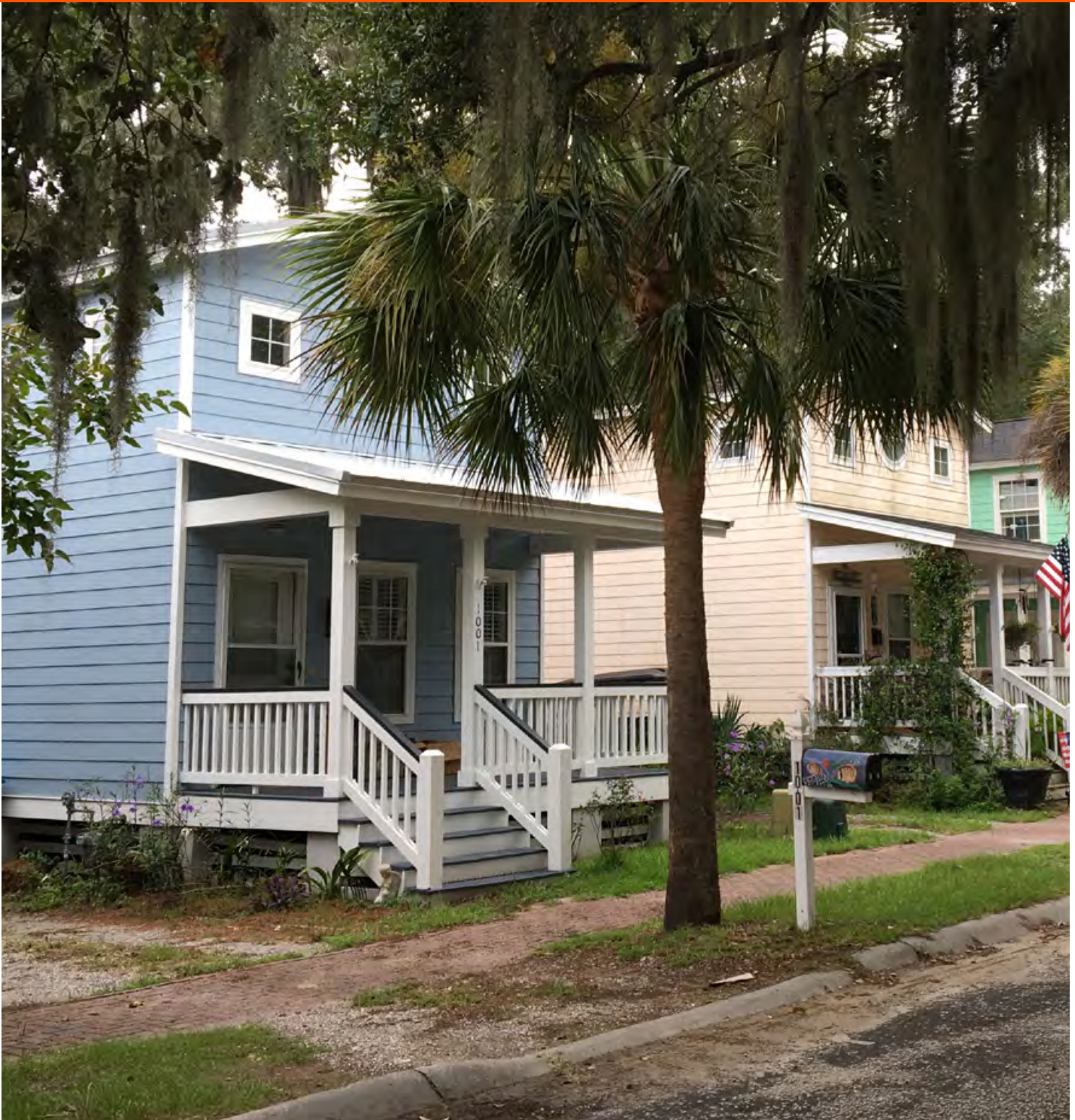
Photo source: Design Workshop
